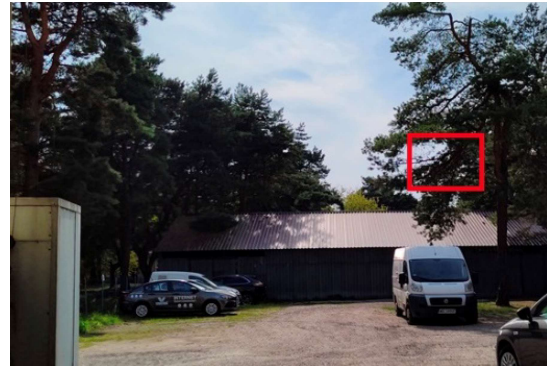
Fig. 6. View from the calibration station location in the satellite direction before tree crown trimming.
